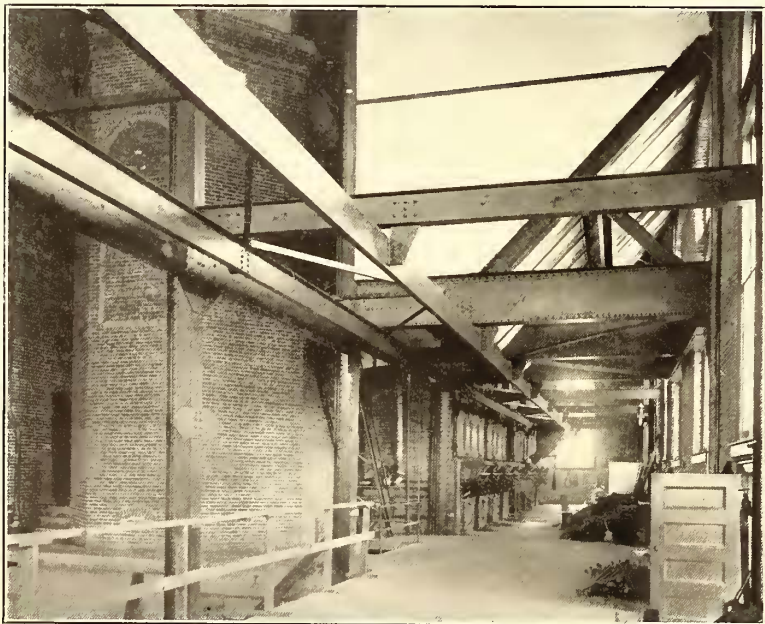
BOILER ROOM, SHOWING FUEL-HANDLING OUTFIT AND STOKERS
