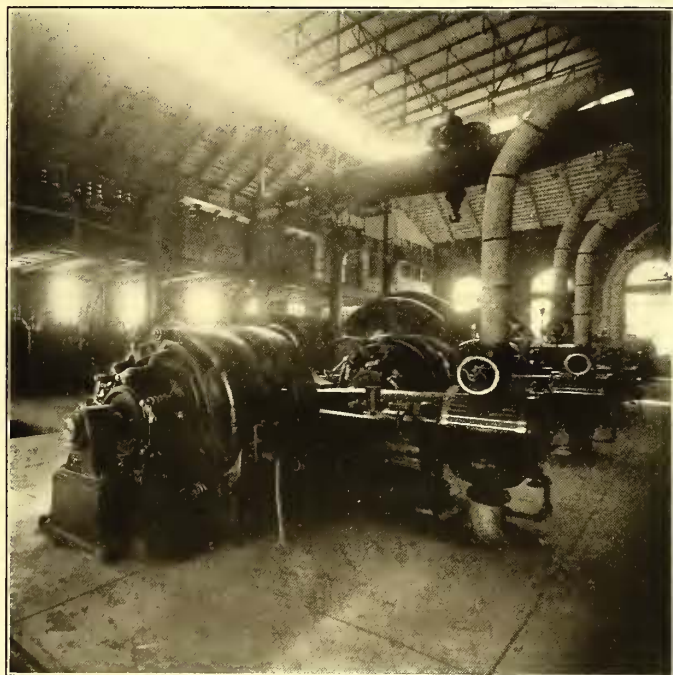
GENERAL INTERIOR VIEW, SHOWING EXCITER SETS
