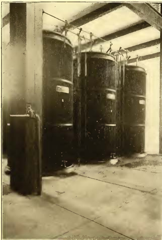
370-KW OIL-COOLED TRANSFORMERS IN MAIN POWER STATION
